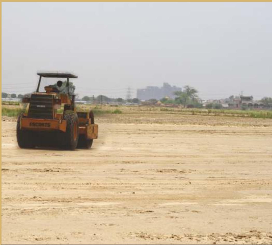
NORTHERN PERIPHERY ROAD (DWARKA EXPRESSWAY) UNDER CONSTRUCTION
